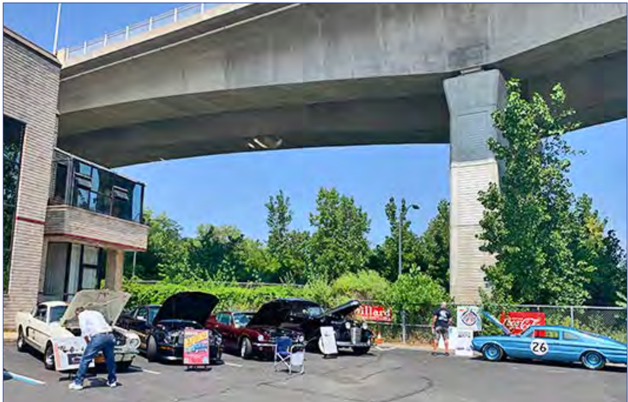
Beneath the Roslyn Viaduct.
