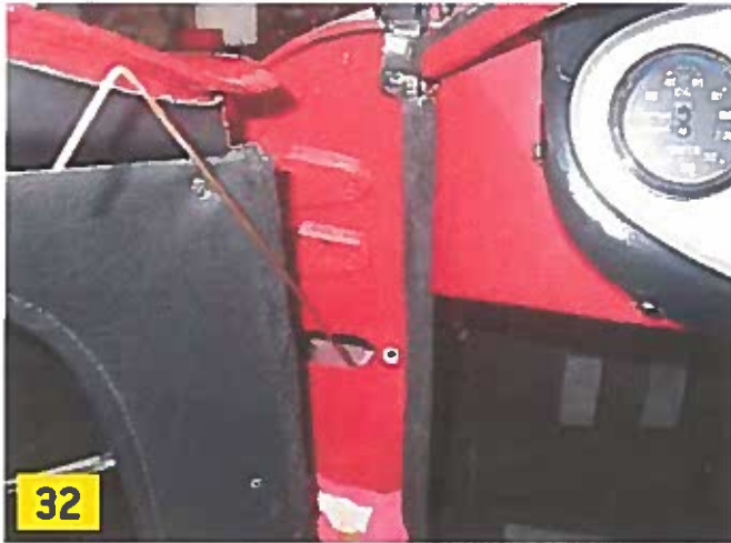
Photo 32: The handle end of the wire used to install a door check on the 100s. This photo was taken during replacement on a finished car.
