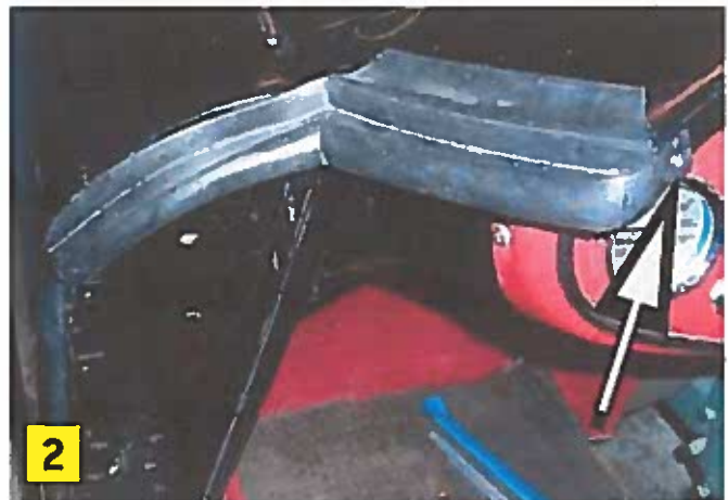
Photo 2: After mounting the seal to the flanges of the shroud and front wing, a #6 trim screw (but with no cup washer) is used to position the flap as shown. This will be hidden by the front of the dash pad.
