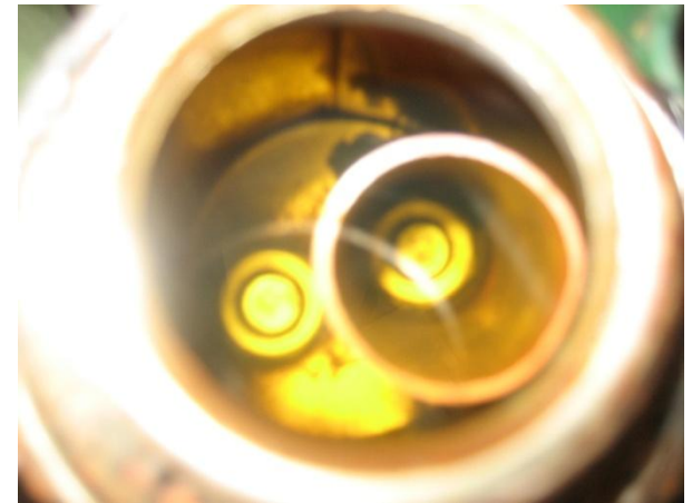
View of top of Hydraulic reservoir
