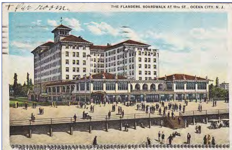
Completed building before fire.
