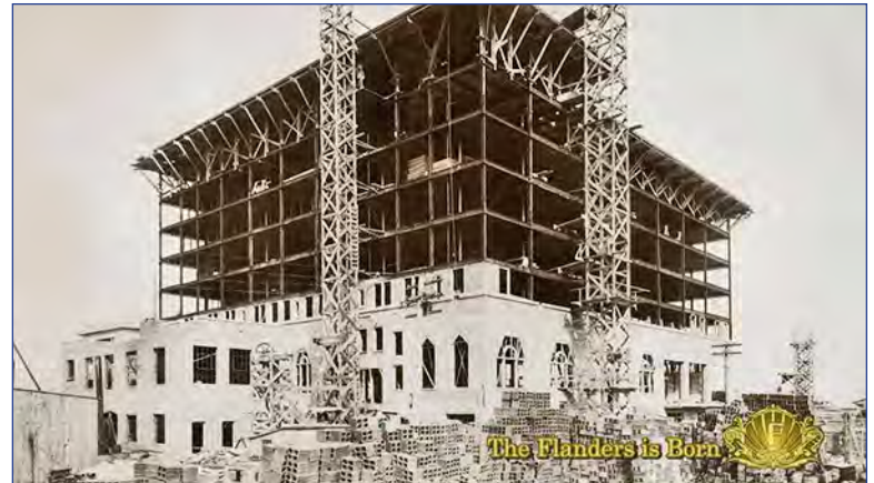
Initial concrete construction.
